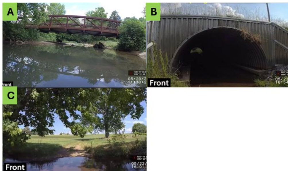
Figure 13: Example images of Road discrete point feature type including bridge (A), culvert (B), and low water crossing (C). Example images may not be from this project.
