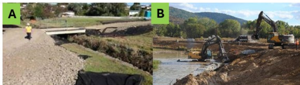
Figure 14: Example images of Construction discrete point feature type including near-channel (A) and in-channel (B). Example images may not be from this project.
