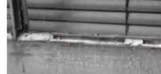
Examples of degraded caulk in poor condition
