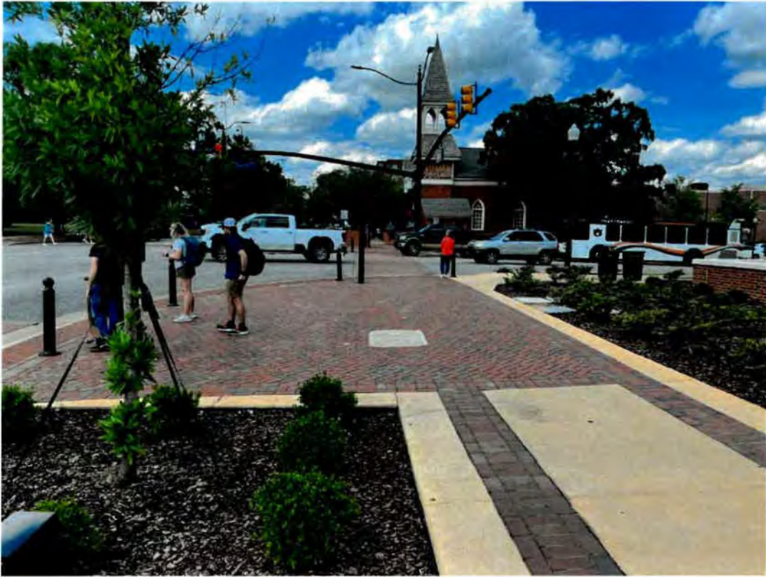
Pervious Paving along S. College St. (Tony & Libba Rane Culinary Science Center- AU Project # 16-370)
