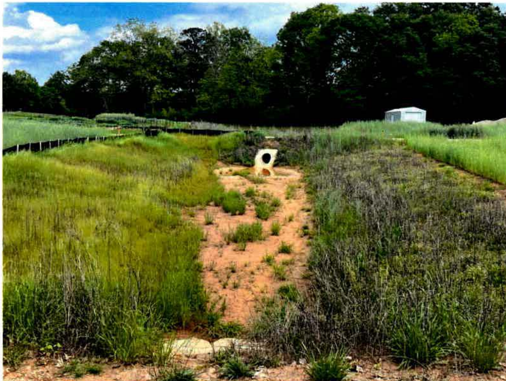
Detention Pond at Transformation Gardens (Duncan Drive Extension and Infrastructure- AU Project # 20-105)
