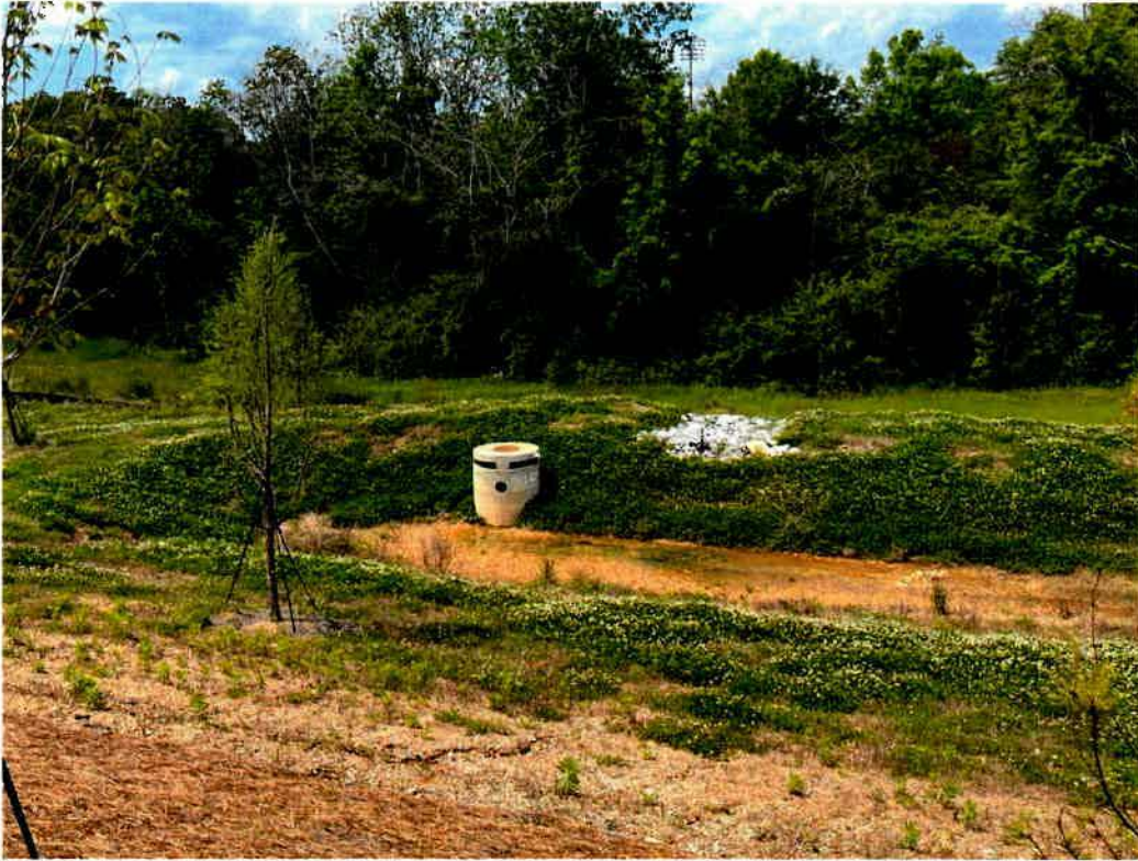
Detention Pond at Chilled Water Plant (Chilled Water Plant- AU Project # 18-444)
