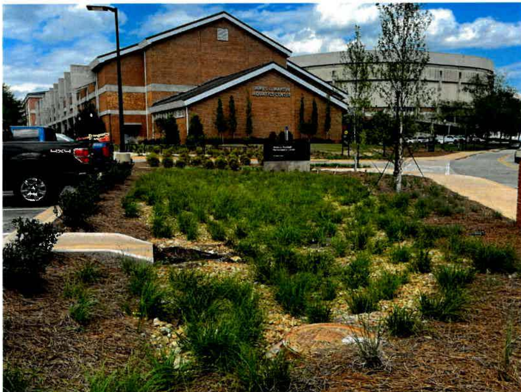
Bioretention at the Football Performance Facility (Football Performance- AU Project # 19-441)
