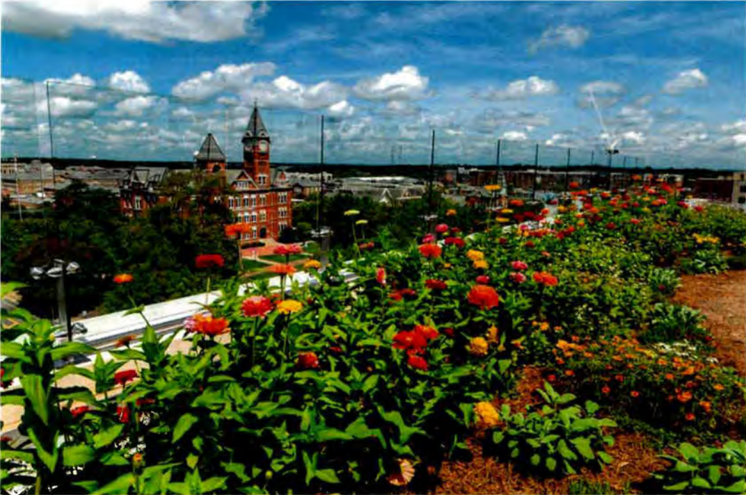
Green Roof at Rane Culinary (Tony & Libba Rane Culinary Science Center- AU Project # 16-370)
