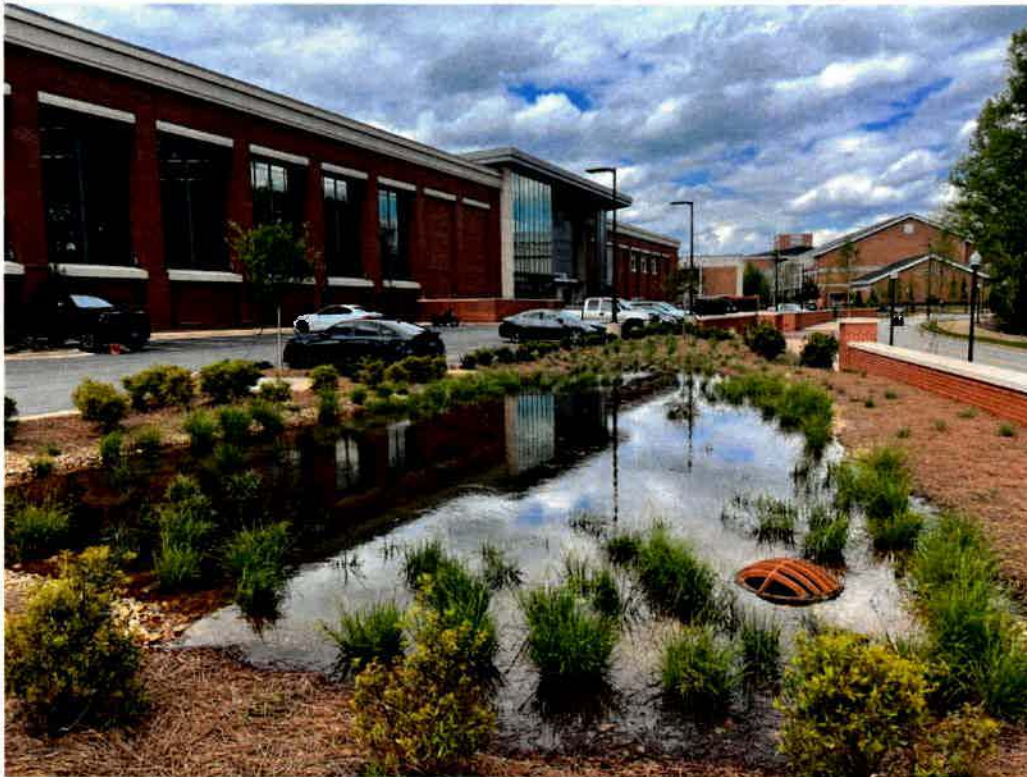
Bioretention and cistern at the Football Performance Facility (Football Performance- AU Project # 19-441)
