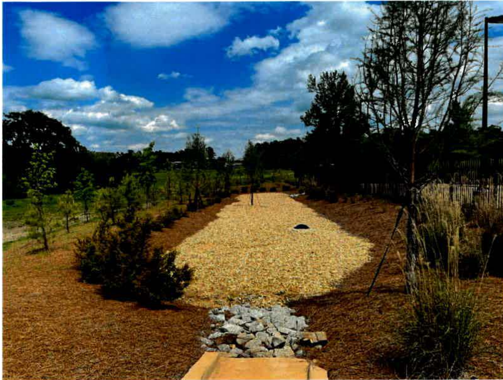
Bioretention at Chilled Water Plant (Chilled Water Plant- AU Project # 18-444)
