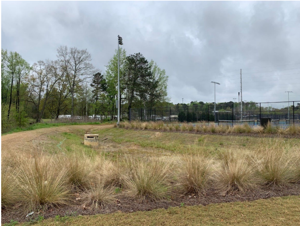
Detention Pond at New Tennis Courts (Football Performance Center Tennis Court Relocation - AU Project 19-441).
