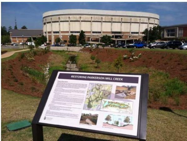
**The Parkerson Mill Creek restoration project** adjacent to the Wellness Kitchen included restoration of over 300 linear feet of impaired stream by establishing a stream floodplain, installing in-stream cross vane structures, and planting deeply rooted native plantings all to stabilize the creek from erosion and improve the water quality.
