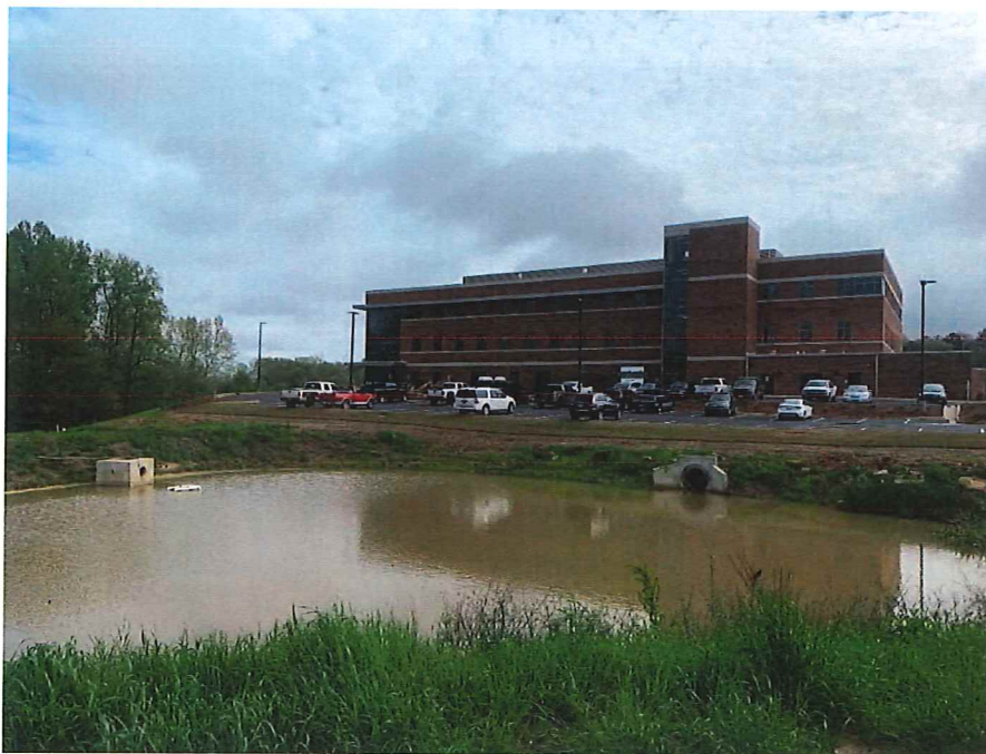
Detention Pond at Auburn Research Park Building 6 (EAMC Facility – AU Project 18-121)
