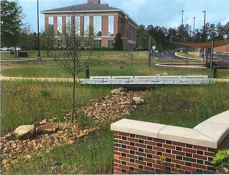
BioRetention at Auburn Research Park Building 5 (Research and Innovation Center - AU Project 18-236)
