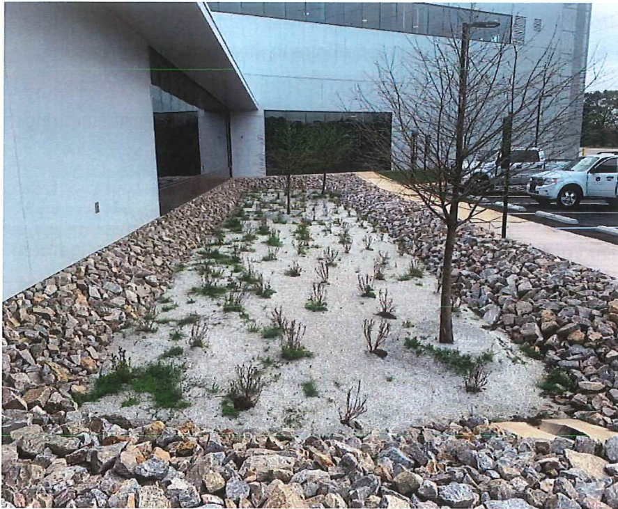
Bioretention Cell at Advanced Structural Engineering Laboratory (AU Project 17-255)
