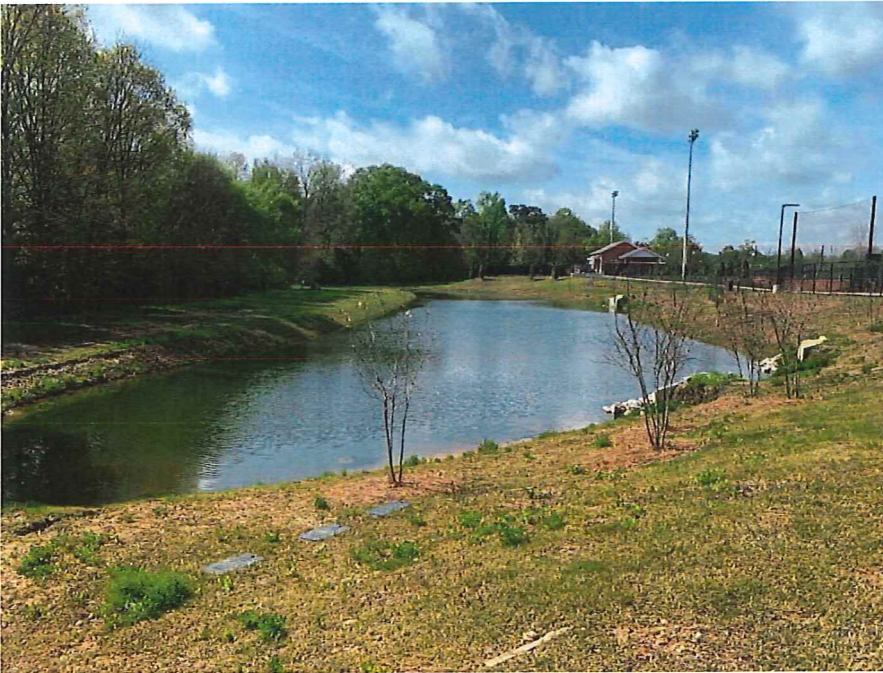
Retention pond at the Campus Recreation SportsPlex (AU Project 18-028)
