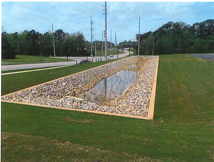
Bioretention Cell at Advanced Structural Laboratory (AU Project 17-255)
