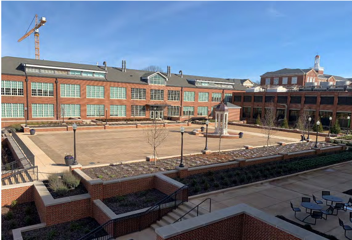
Green Roof at Brown Kopel Engineering Student Achievement Center (AU Project 15-157)
