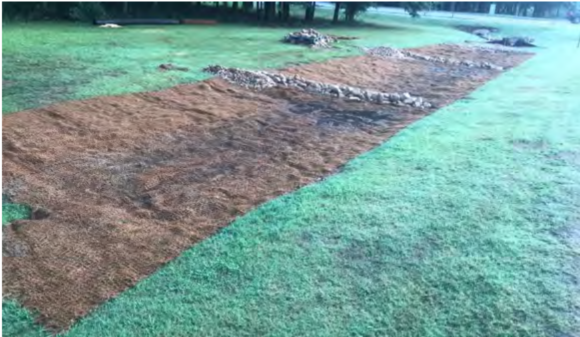
Figure 1: Finished construction of the downstream end of the project site.
