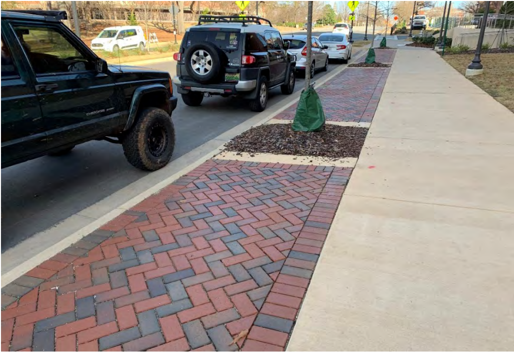
Pervious paving at the South College Street Parking Deck (AU Project 18-071)
