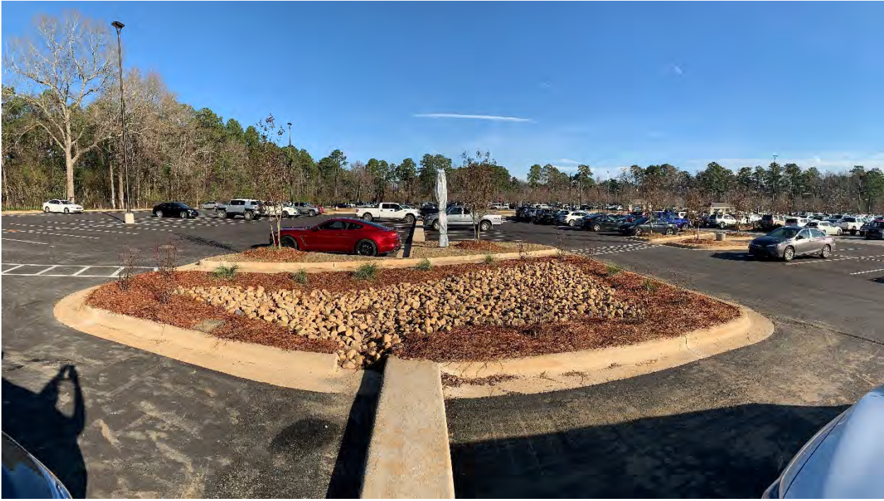
Bioretention at the West Campus Parking Expansion (AU Project 19-037)
