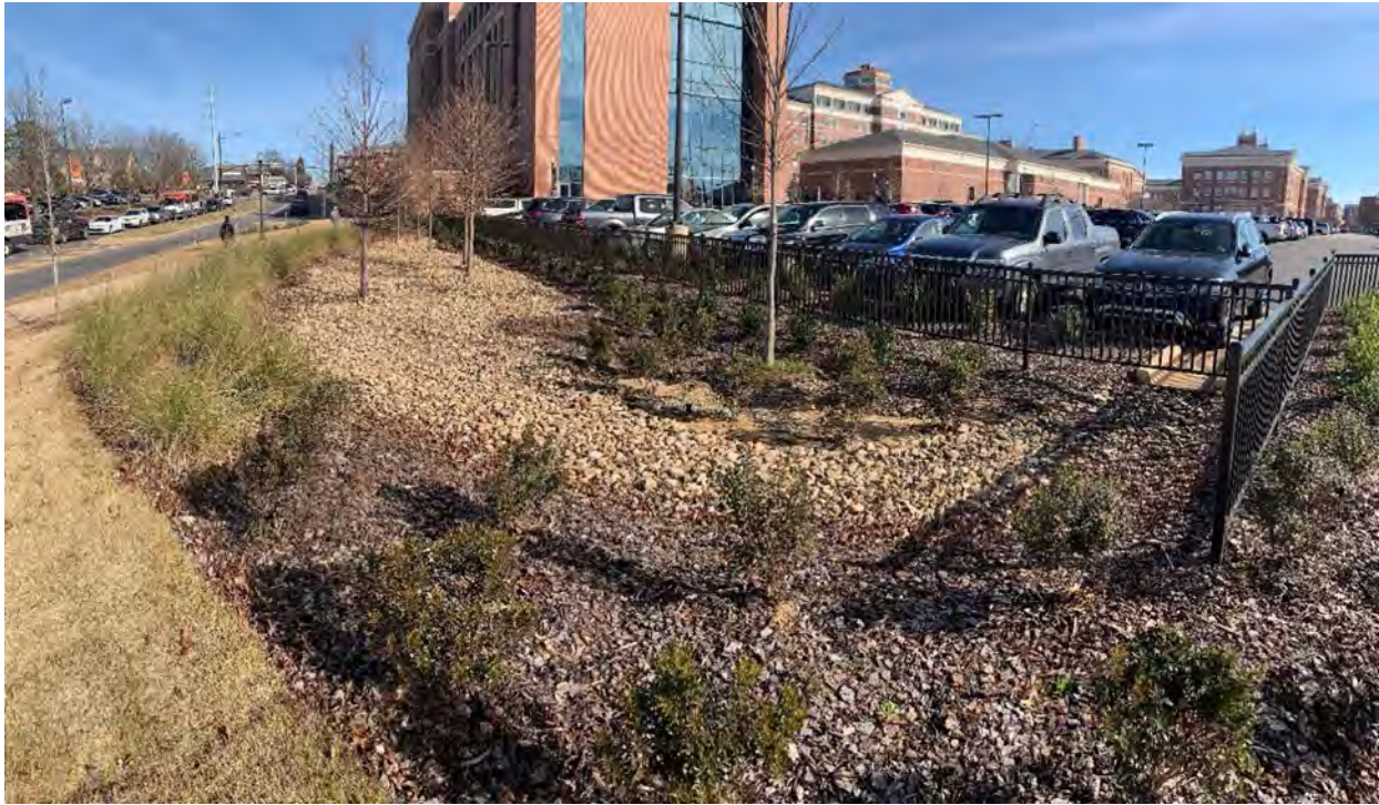
Bioretention Cell at Horton Hardgrave Hall (AU Project 14-044)
