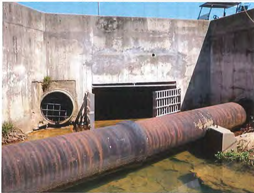
General Location: Coliseum (smaller round pipe on the left)
