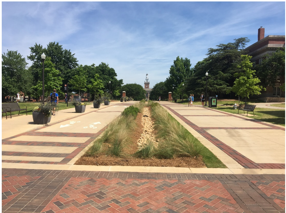
Bio-retention at the Mell Concourse Center (AU Project 15-311)
