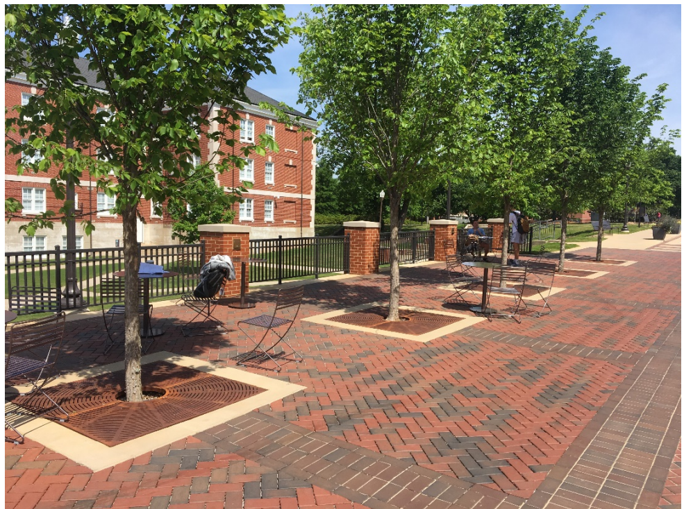
Pervious paving at the Mell Concourse Center (AU Project 15-311)
