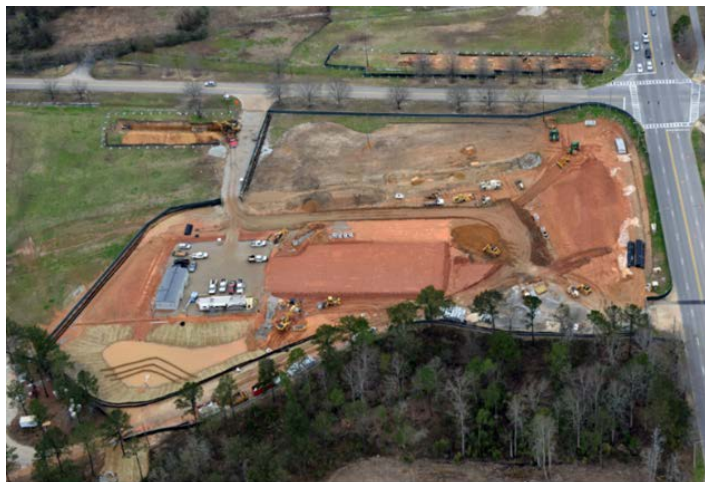
Health Sciences Sector site under construction utilizing sediment pond
